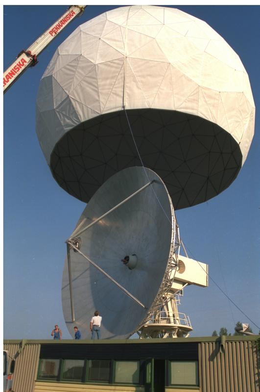
Figure 4.11: Single dish antennas - Metsähovi Radio Observatory, a 14-m antenna in Kirkkonummi, operated by Helsinki University of Technology
